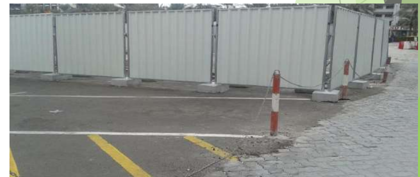
4.CONSTRUCTION BOUNDARY FENCE
